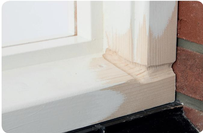
**Tip:** Use the blunt side of a screwdriver to identify the rot spots.
