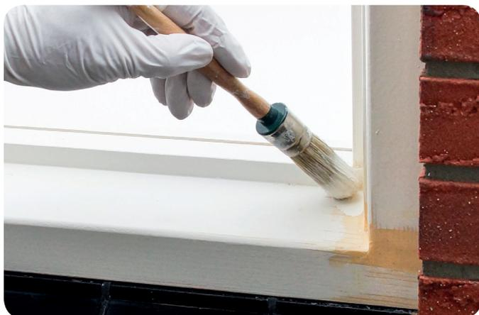
**Tip:** Use our Fine Surface Filler on top of the cured Wood Filler. This will ensure an extra smooth result. Make sure to sand first!
